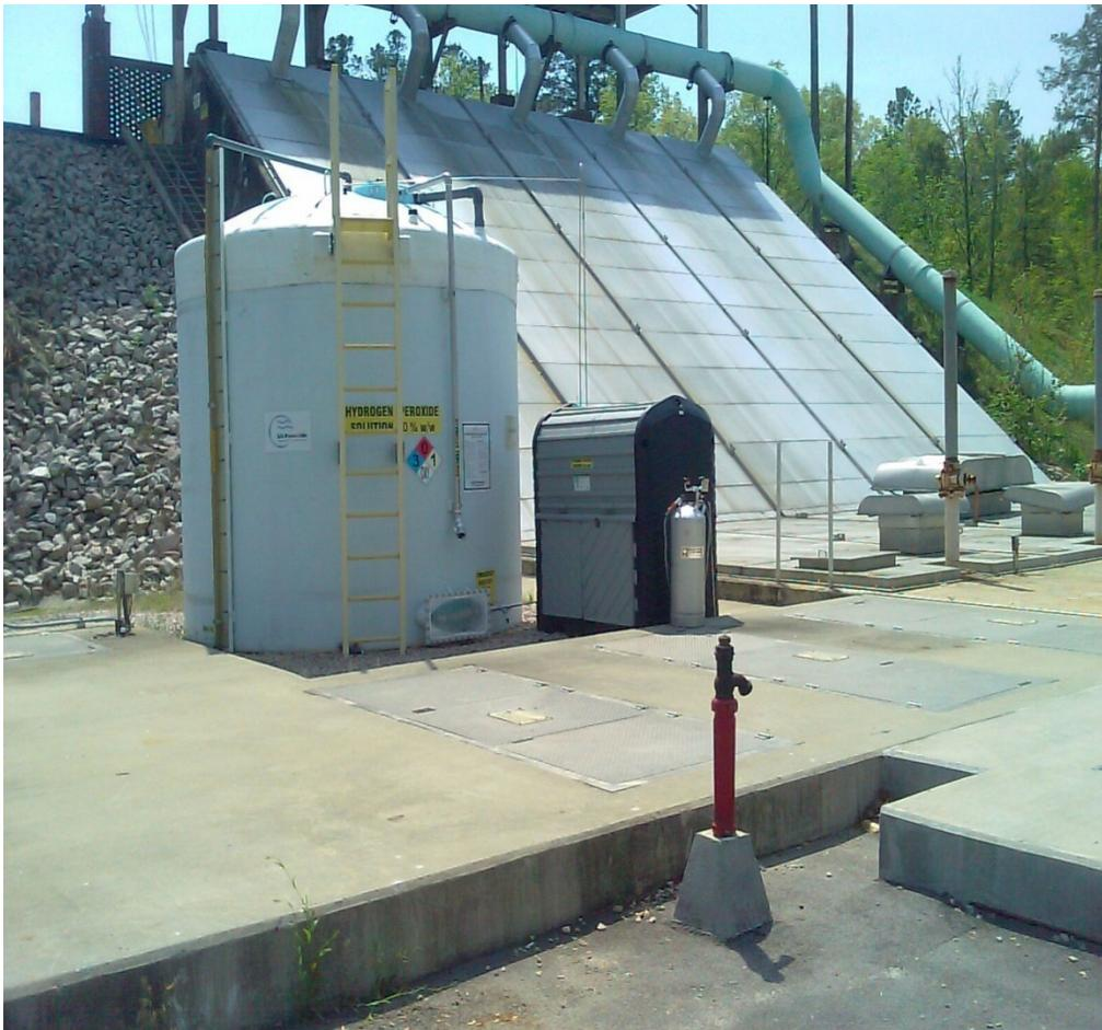
**Figure 4. Hydrogen Peroxide System Installation at Walnut Creek Lift Station**
