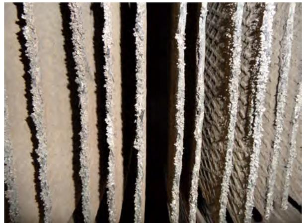
**Figure 2. Asbestos Cement Board (ACB) fill**
