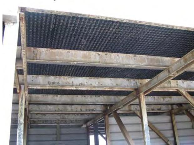
**Figure 28. Structural supports after peroxide cleaning showing algae substantially bleached and removed.**
