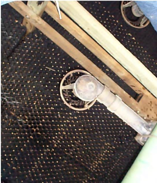
**Figure 35. Fouling is not readily apparent on cursory inspection looking down from spray nozzles.**
