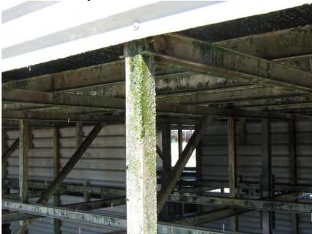
**Figure 27. Structural supports prior to peroxide cleaning showing some green algae buildup.**
