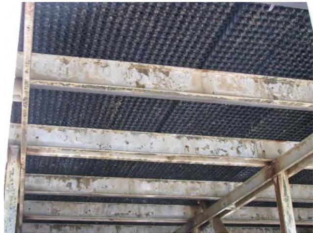
**Figure 24. Tower pack after peroxide cleaning.**
